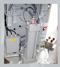
This  $\emptyset5" \times 32.00"$  stroke actuator has a  $\emptyset2"$  rod and is equipped with full stroke postion indication to determine percentage of valve positioning.
